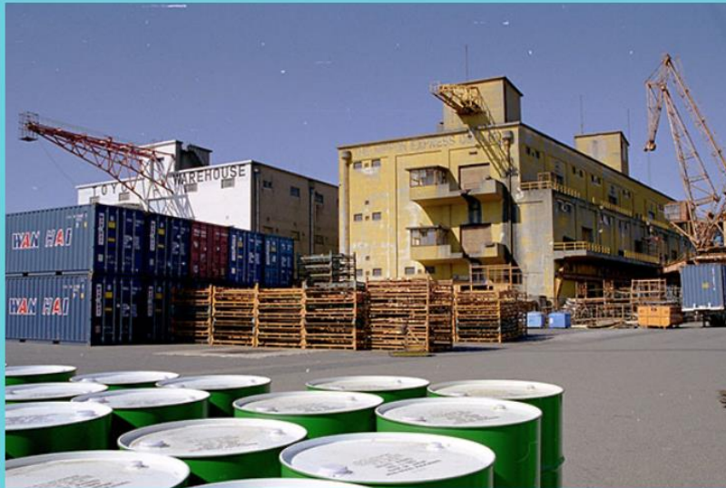
Garden pier in the port of Nagoya Warehouse No.20 (© Muto Isamu [N-mark])
